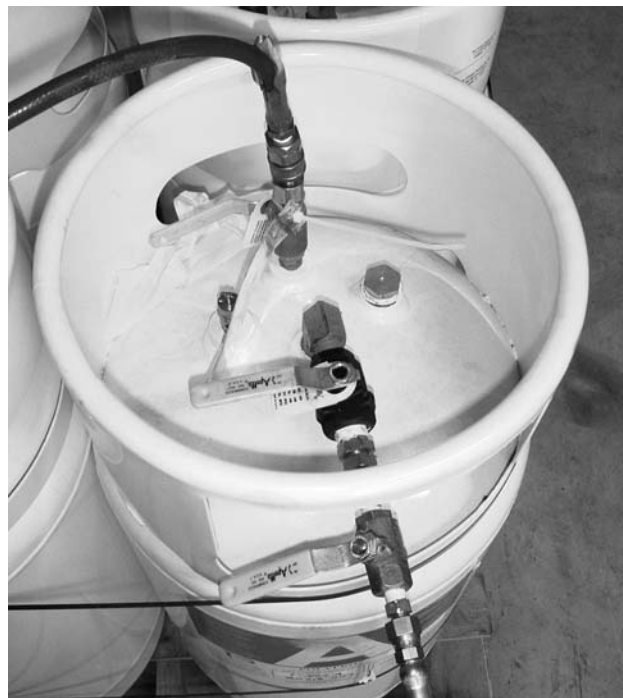
When changing cylinders make sure all chemical valves and nitrogen valves are closed.
